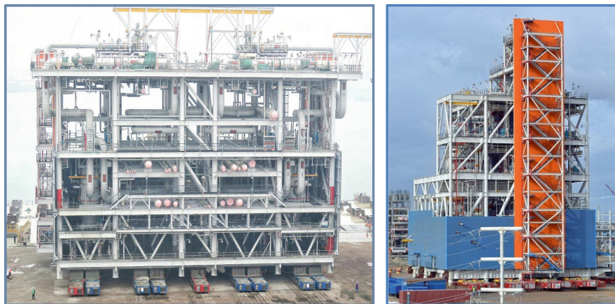
Fig. 3. Modules for the construction of the LNG plant. Photo by PJSC NOVATEK
