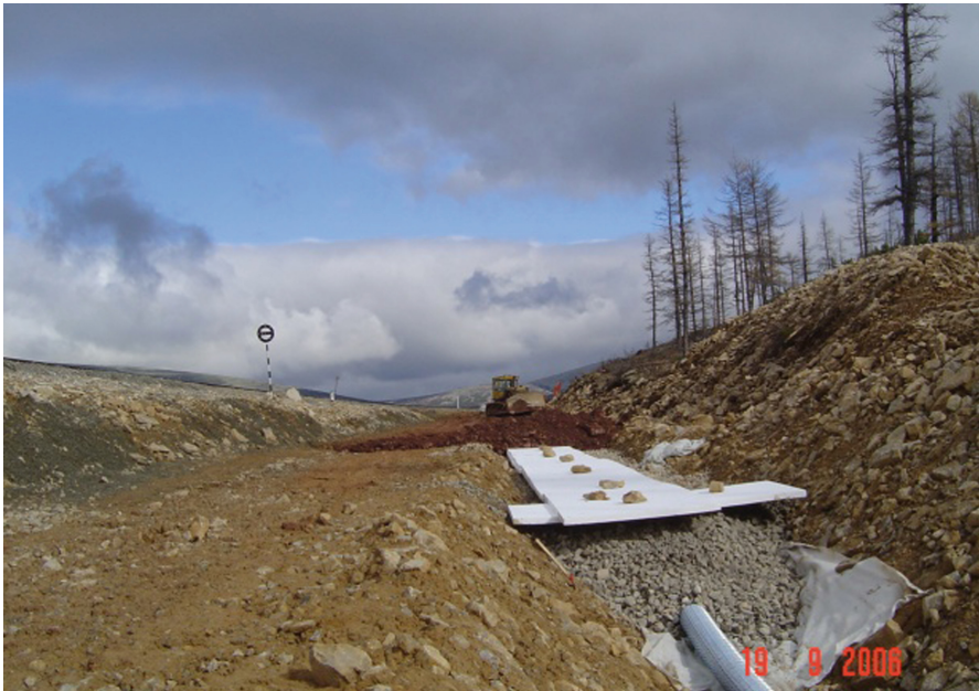
Fig. 6. Installation of deep warmed drainage in conditions of underground water strikes and thermal karstification
