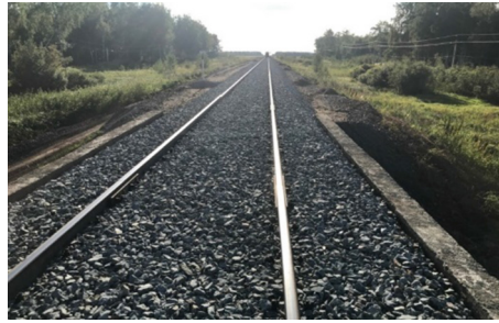
Fig. 5. Part of the railroad track (ballasting phase) after repositioning of the track to the project values with an electric ballast vibrator equipped with ACS-3D utilizing a satellite reference net
