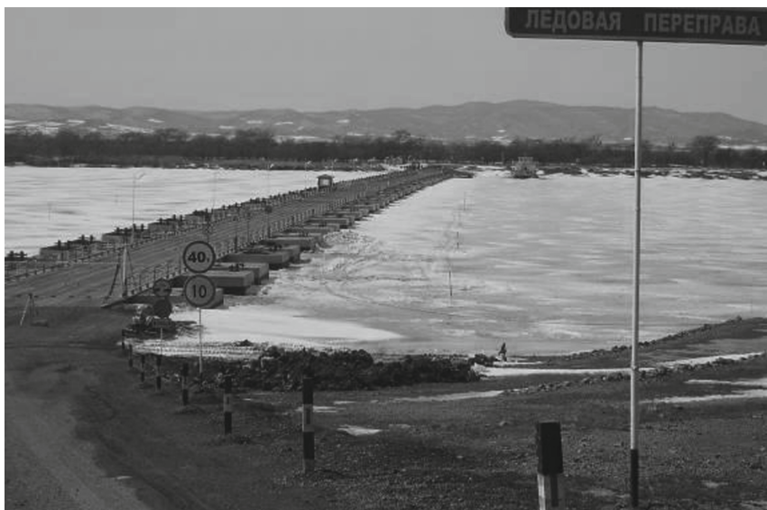
Fig. 1. General view of the ice crossing reinforced with metal pontoon structures
