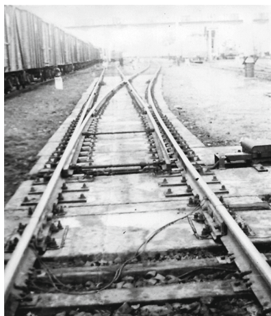
Fig. 1. General view of the switch on the slab base
