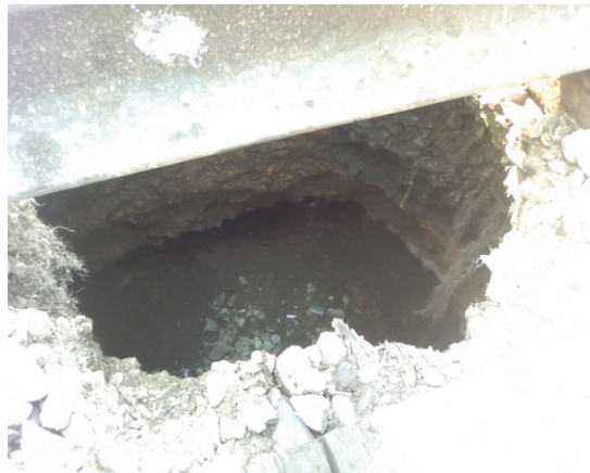
Fig. 4. Injected ice in collapse sinkhole of rail seat (in May)
