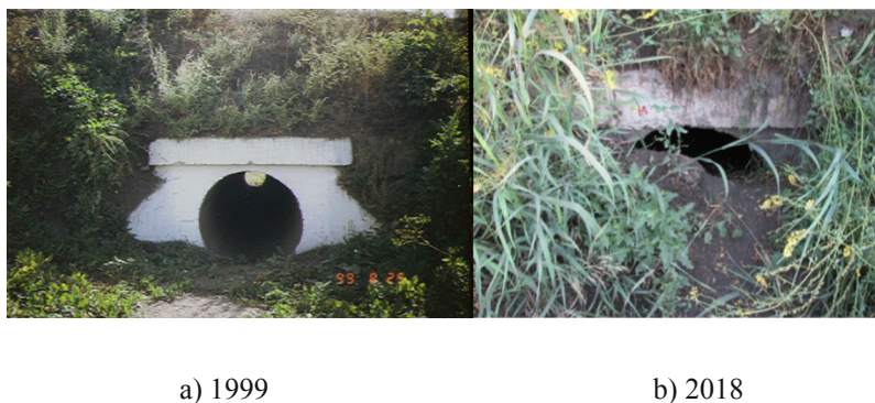
Fig. 2. Culvert pipe and its technical condition in 1999 and 2018.
